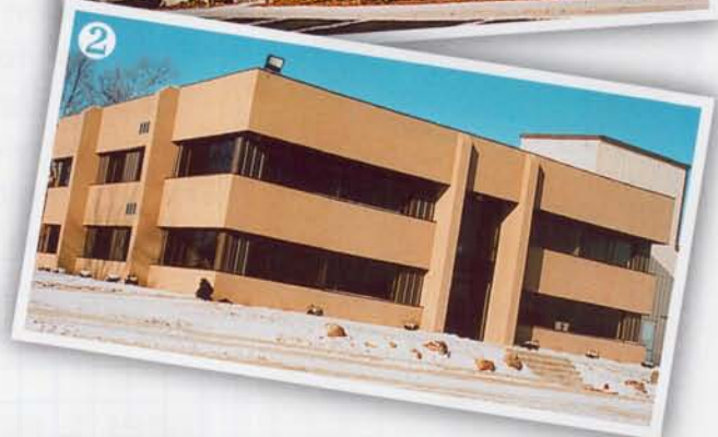
1 Office warehouse structure.
